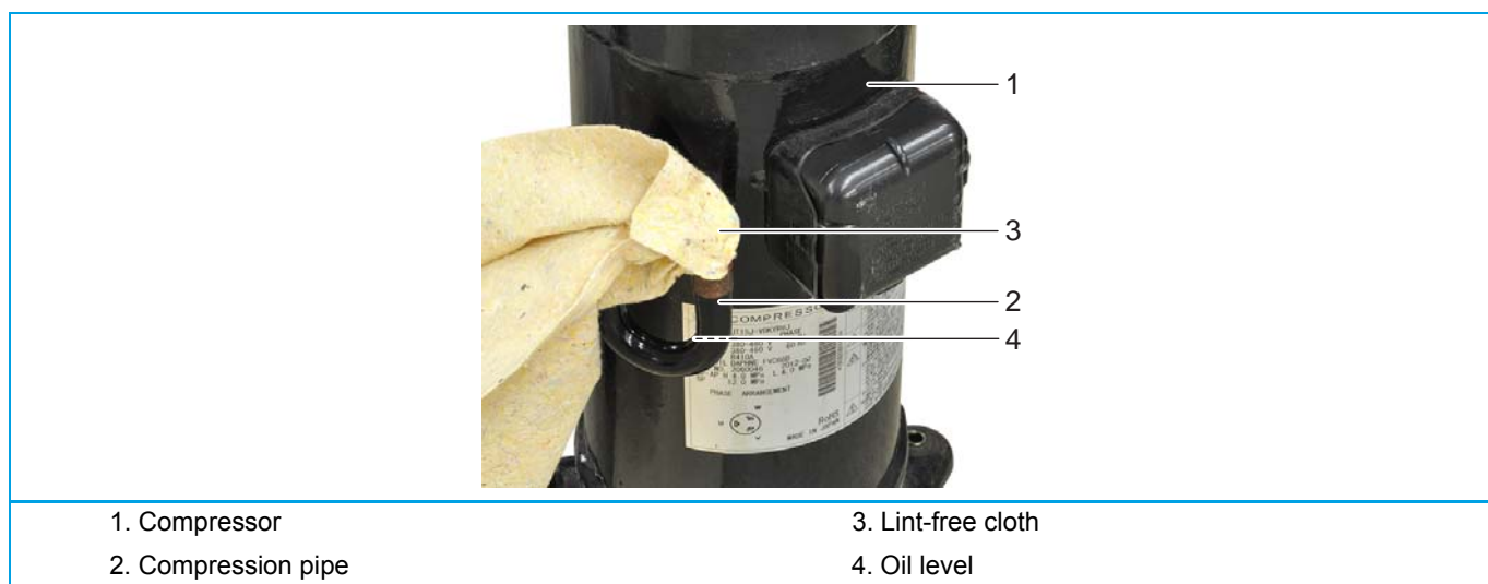
Figure 74 - Installing a new compressor - 2
