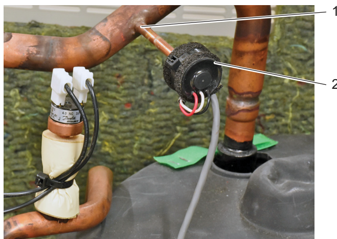
Figure 3-19: Removing low pressure sensor
