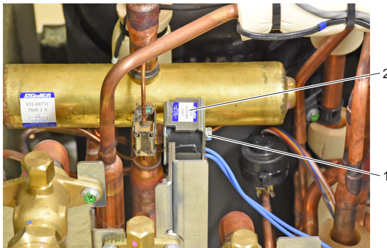
Figure 3-10: Removing the 4-way valve coil
