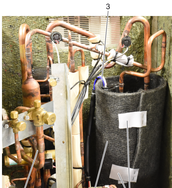
Figure 3-7: Removing the compressor jacket
