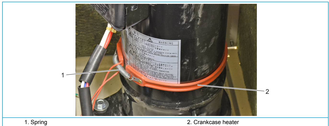
Figure 3-13: Removing the crankcase heater
