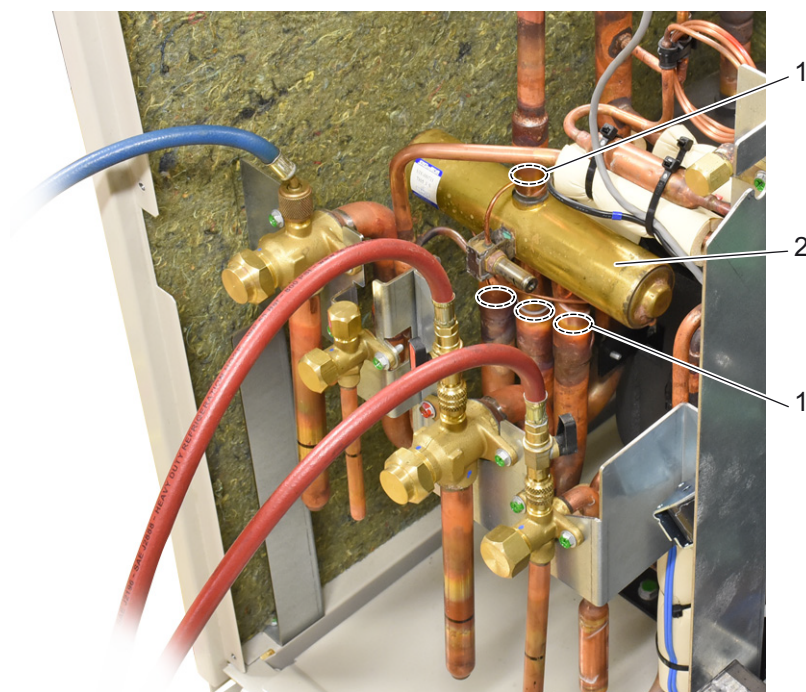
Figure 3-9: Removing the 4-way valve body
